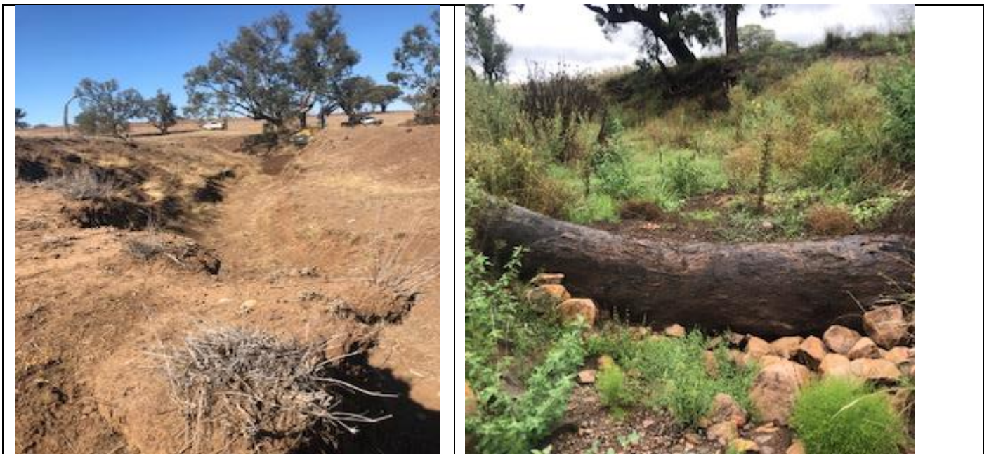
Water Gully Jobys Hill reach Structure 2 – L-October 2019, R-March 2021
